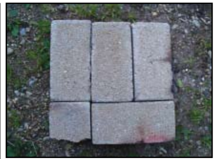
Brick stove layer 1
